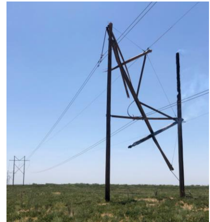
Figure C.1: Failed H-Frame
