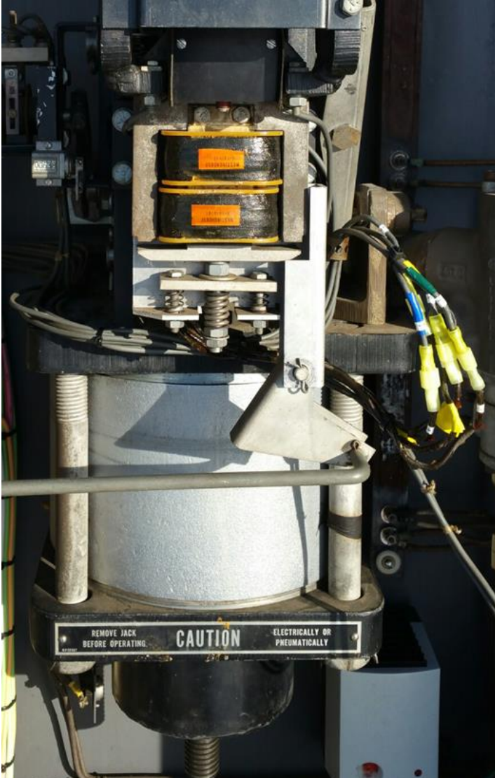
Figure 3: Trip Coil Assembly
